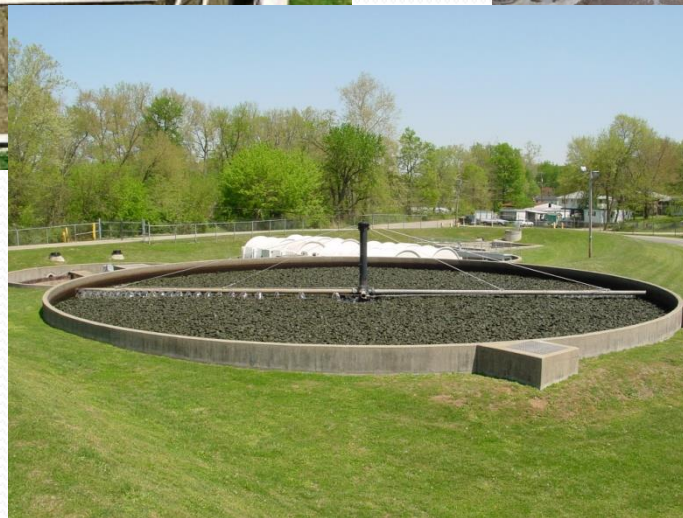
Trickling Filter
