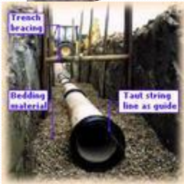
Laying New Sewer Pipes
